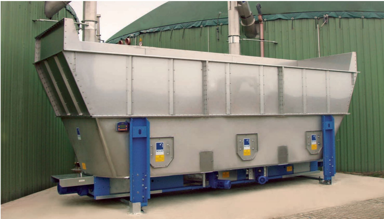
Solid matter dosing unit model 500 with two 3-piece screw sections for feeding two fermenters
