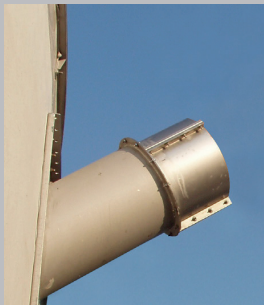
Silo connection plate for fermenter screws
