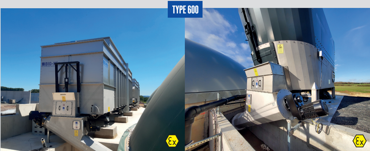
Fermenter screws TYPE 600 according to ATEX feed the fermenter directly. Both units are equipped with a slide opening for this purpose.
